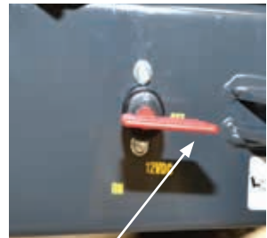
Main switch – OFF
