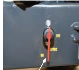
Main switch – ON
